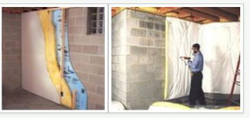
Continuous Insulation: If the basement is a heated space, then insulating the walls is suggested.
