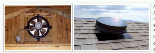
Attic Exhaust Fans: Attic exhaust fans aren't necessary if your attic is well sealed and insulated. These fans only need to run if the heat is excessive (100 degrees) or if you access the attic space often. There are
