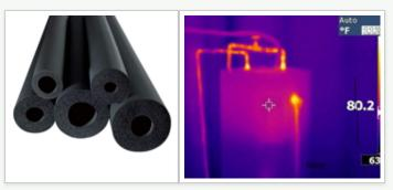
Foam sleeve type insulation works well on water heating pipes. The first 6 to 10 feet closest to the water heater provide the most benefit to insulate.
