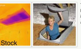
Typically an uninsulated attic hatch is one of the biggest leaks in a home. These should be covered with a rigid board insulation box, insulated tent or dome. If attic access is tight an attic tent may fit better for an attic pull down.
