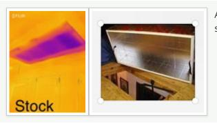
A Thermodome is a good way to insulate over a pulldown stairway.
