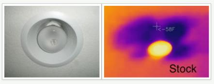
Typical Air Leakage at Can Lights: Recessed lights should be IC (Insulation Contact) rated in order to have insulation installed over them safely.
