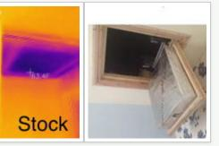
Typically an uninsulated attic hatch is one of the biggest leaks in a home. Insulate the hatch to your attic or crawl space.
