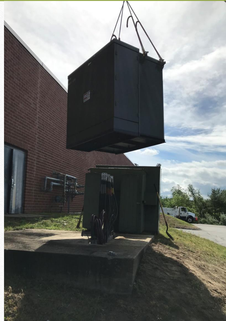
New transformer being set into place...
