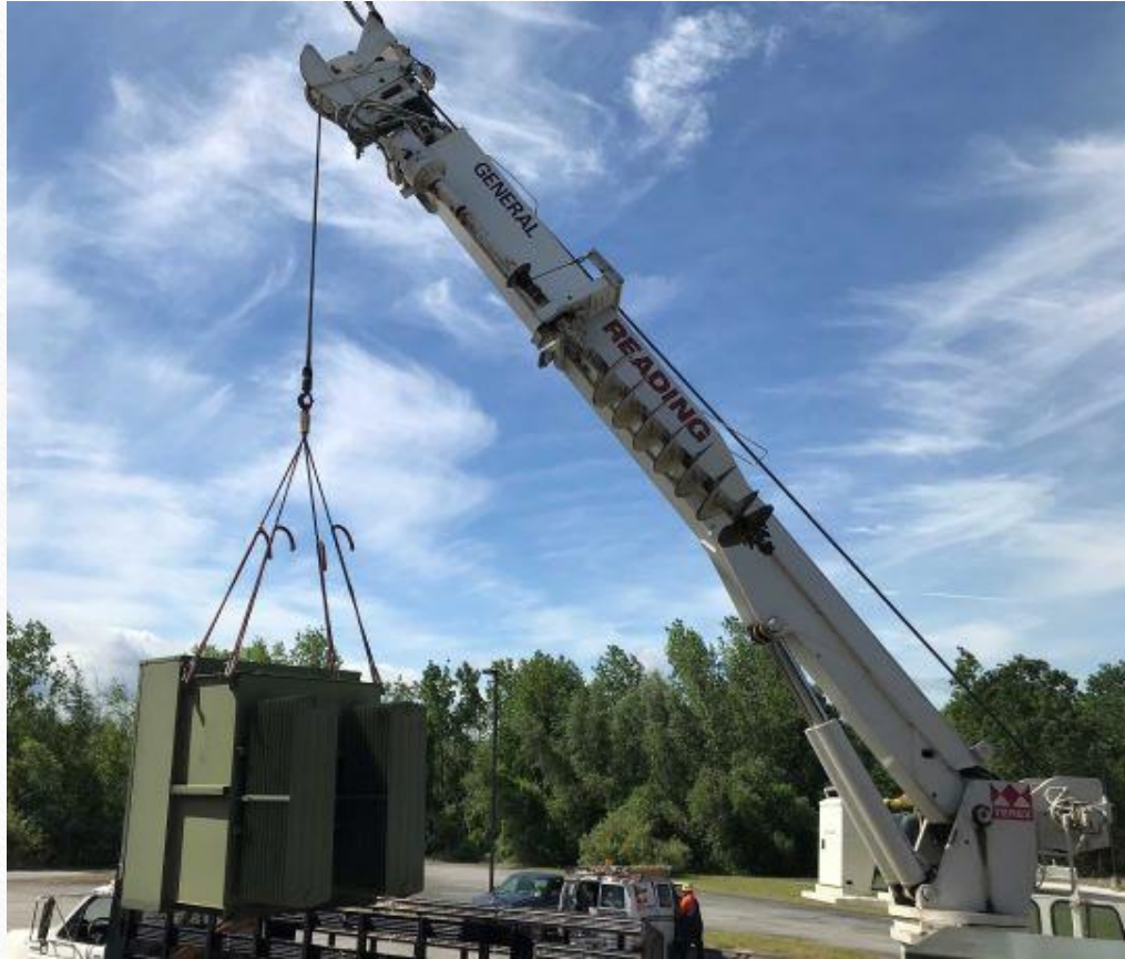
Old transformer being removed . . .
