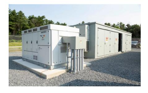
Existing 5 MW / 10 MWH system at Station 3 (profitable for RMLD)
