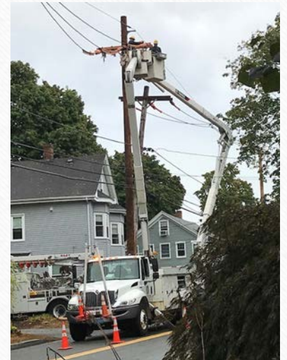
Installation of Scada-Mate Switch on Ash Street, Reading
