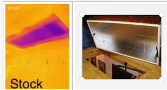
A Thermodome is a good way to insulate over a pulldown stairway.
