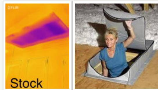
Typically an uninsulated attic hatch is one of the biggest leaks in a home. These should be covered with a rigid board insulation box, insulated tent or dome. If attic access is tight an attic tent may fit better for an attic pull down.
